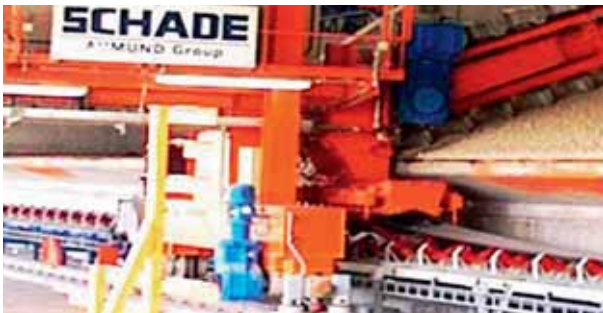
Discharge via impact idler table
