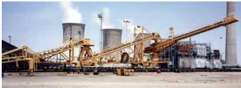
Fig. 4 Stacker with by-pass system
